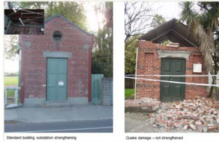
Figure 19: Substation Damage Comparison
