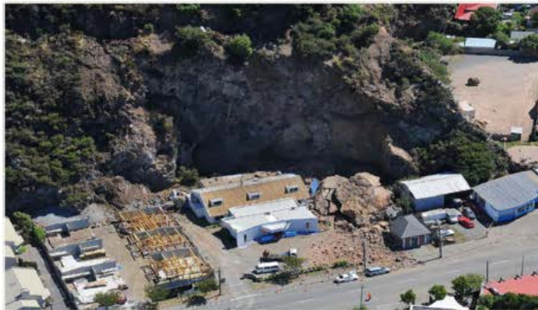
Figure 20: Substation Damage from Bolder - Wakefield Avenue
