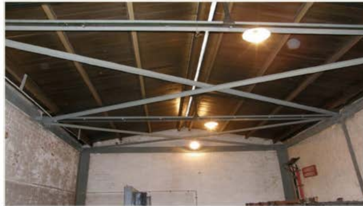
Figure 27: Substation Strengthening - Steel Framing
