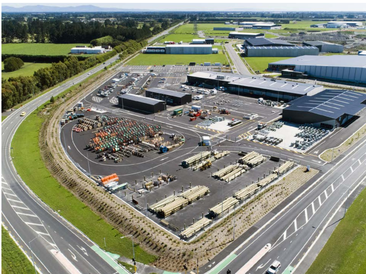
Connetics' new base at Waterloo Business Park.
