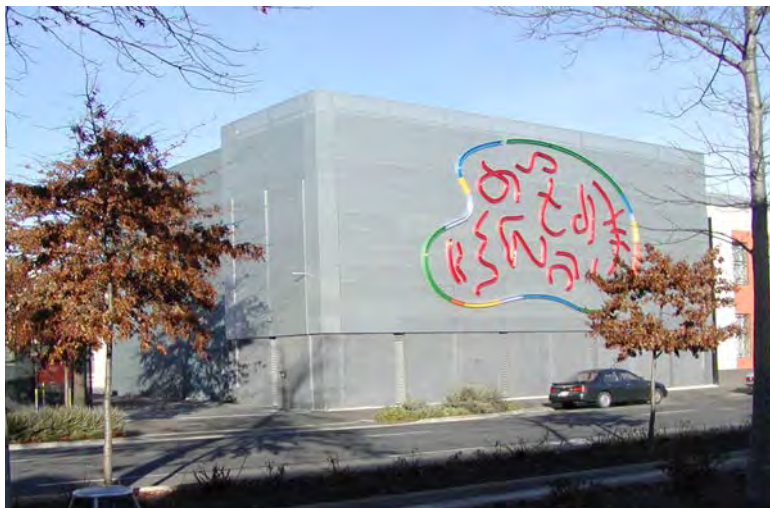
Armagh zone substation, with its neon ‘Nebula Orion’ artwork, contains an ‘outdoor’ 66kV structure.
