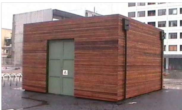
Network substation refurbished as a standalone building after being part of a larger customer building that was demolished due to earthquake damage.
