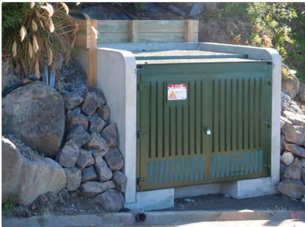
A recently developed kiosk with precast concrete sides, designed to be embedded into a hillside.
