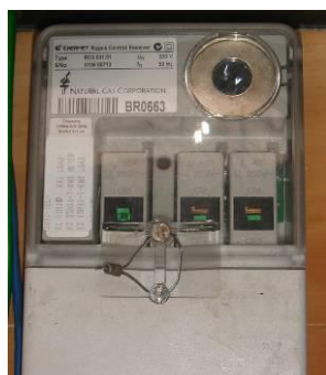
Modern Enermet R03 ripple relay (with Telenerg coding)
